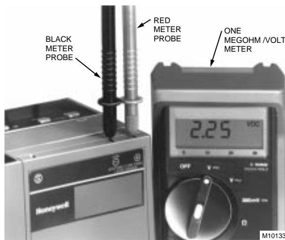
Fig. 9. Measuring voltage flame signal with 7800 SERIES controls.
